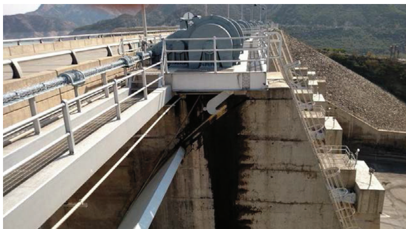
Figure 4. Significant leakage of grease from the gate wheels
