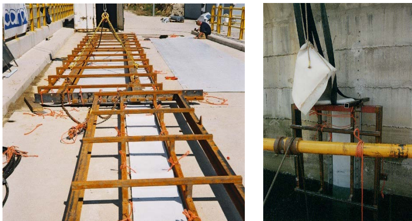
Figure 4. Frame used as template for drilling holes and for correct positioning of the supporting and waterproofing layer forming the Carpi external waterstop.
