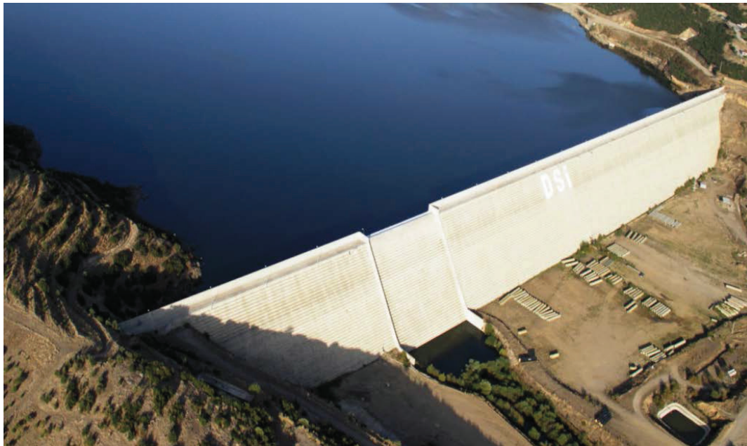
Figure 5. A general view from Beydag dam.
