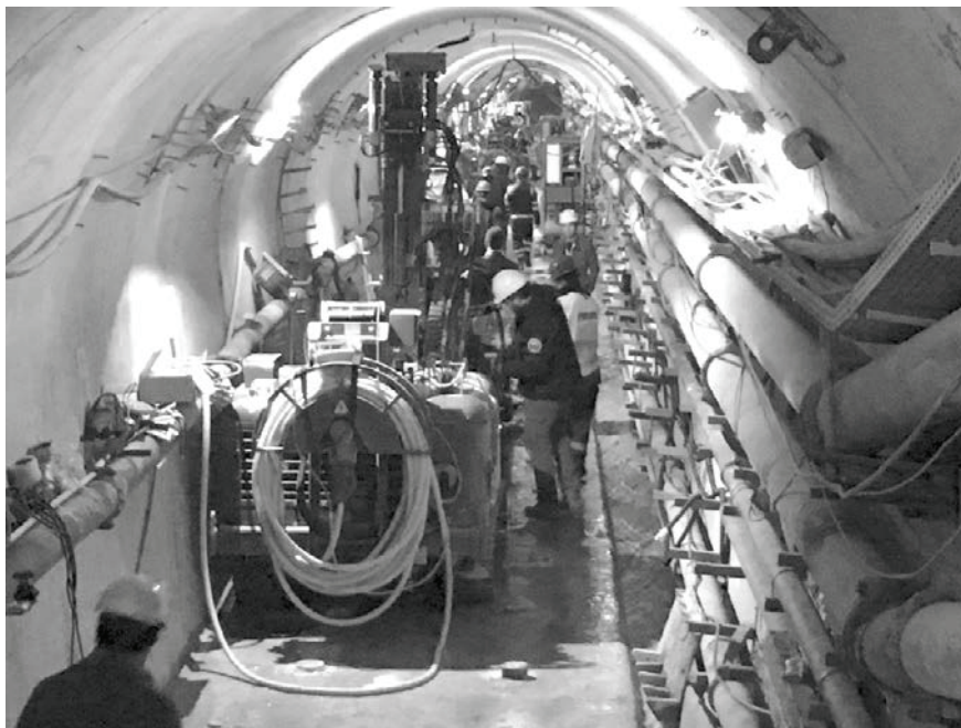
Figure 5. Drilling equipment in the Grouting Gallery (Drill Rig SM5)
