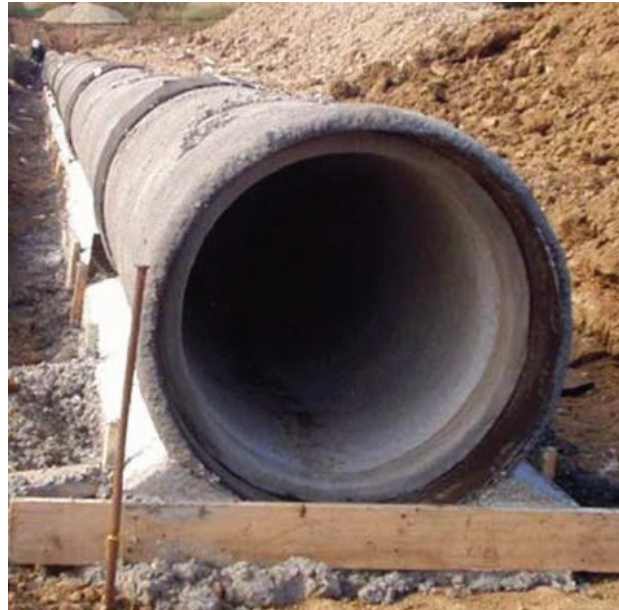
Figure 7. Precast concrete conduit with concrete cradle support (retrieved from FEMA, 2005)
