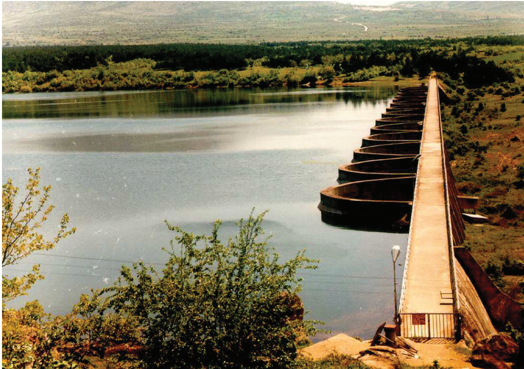
Figure 8. Pripep dam, constructed in 1967, the unique buttress dam in R. Macedonia
