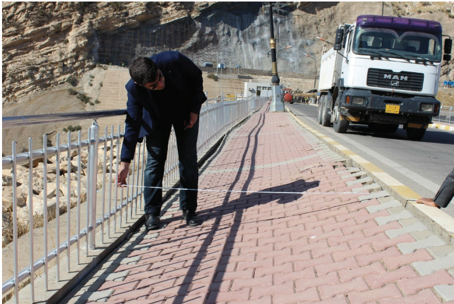
Figure 12. Depression near the downstream longitudinal crack
