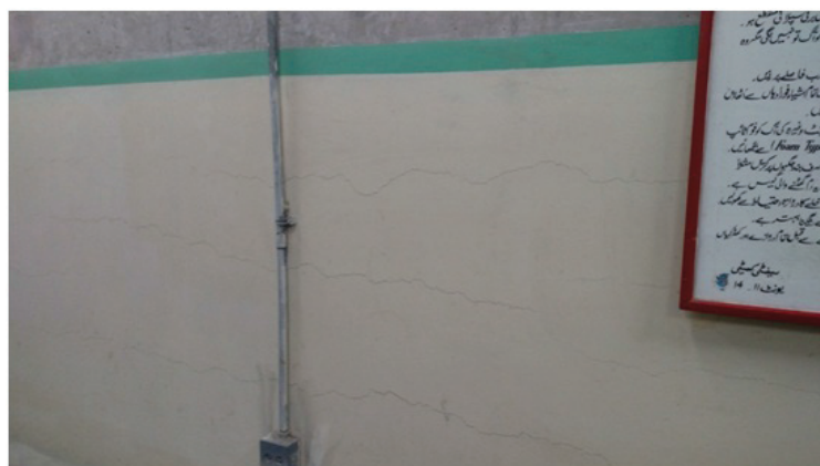
Figure 9. Horizontal cracks in Downstream Wall
