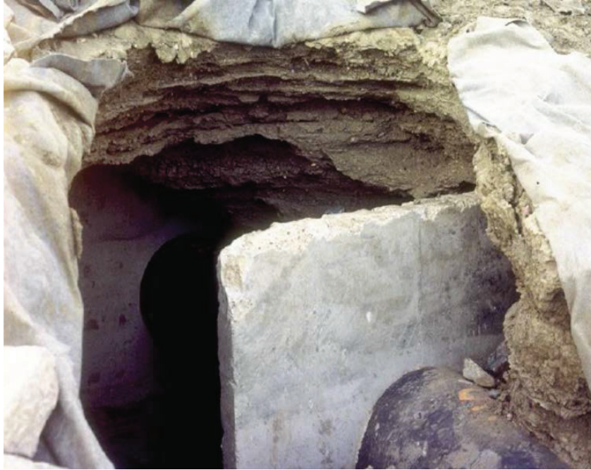
Figure 5. Formation of caverns due to erosion of the backfill adjacent to the anti-seep collars at the upstream end of the conduit (retrieved from ASDSO, 2018)
