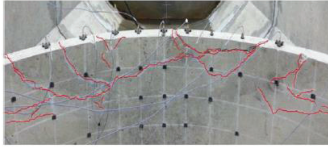
Figure 5. Views of the generated cracks and fractures
