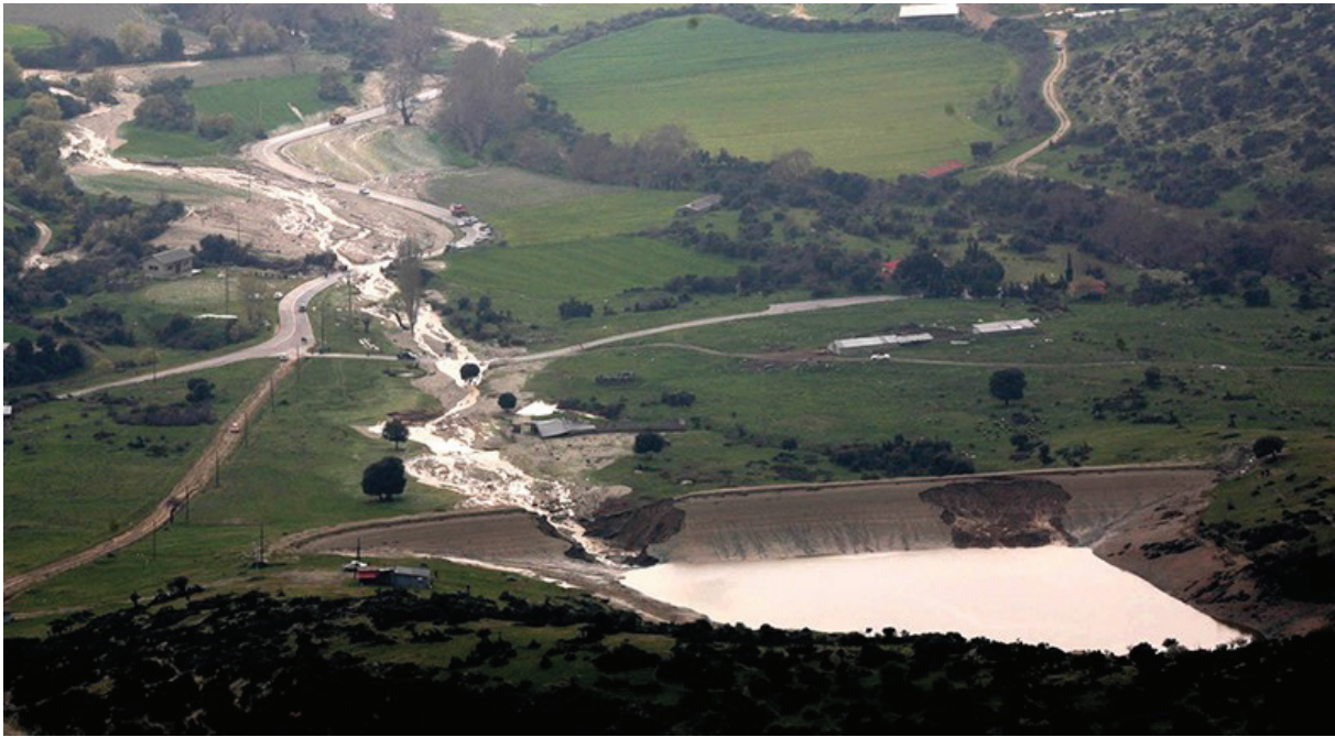
Photograph 5. Sparmos Dam failure, 2016 (Dounias et al, 2017) Photo by Eurokinissi
