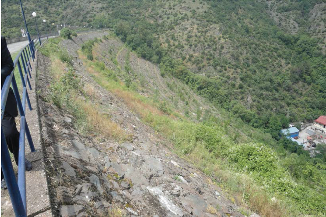
Figure 7. Downstream slope of Tikvesh dam, constructed in 1968, the highest embankment dam in ex Yugoslavia
