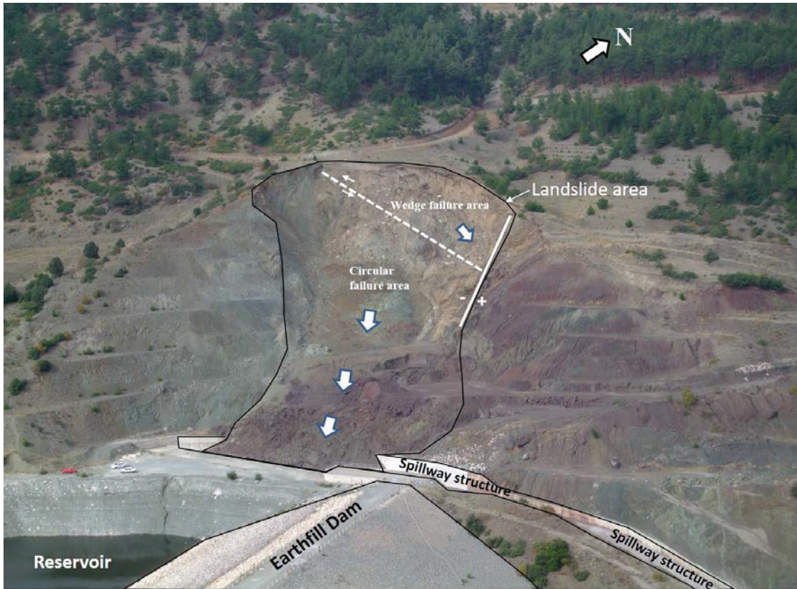
Figure 4. View of spillway landslide area of Beylerli dam.
