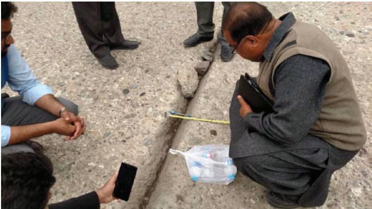
Figure 11. Erosion and Opening of Concrete Panels at Dal Darra Weir
