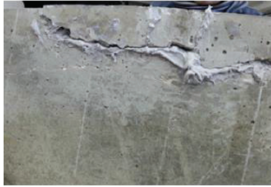
c) Putting in the removed concrete pieces
