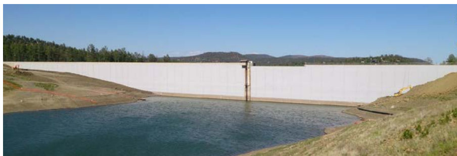
Figure 8. Upstream face of Grindstone Canyon RCC dam after completion of the waterproofing works.
