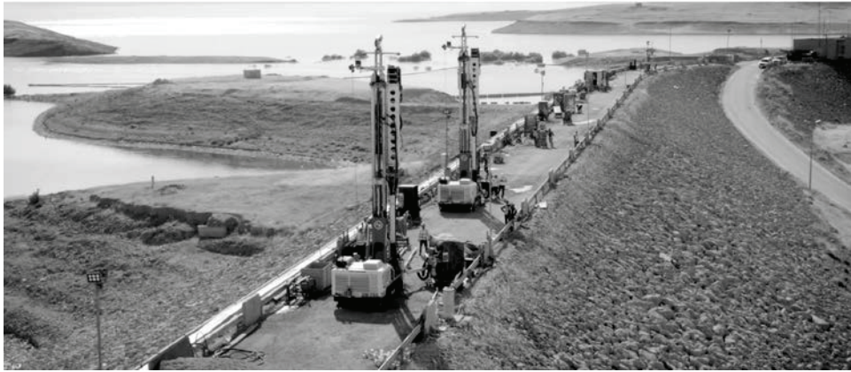
Figure 6. Drilling Equipment at the East Left Bank (Drill Rig SM16)
