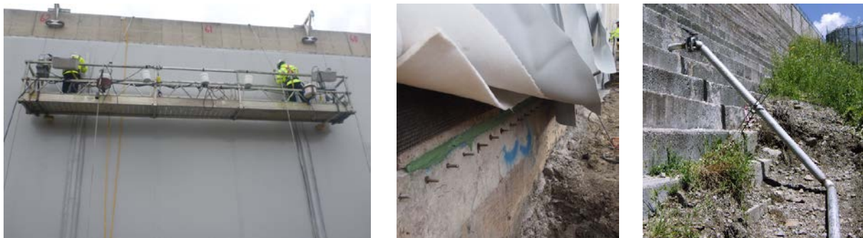
Figure 7. (Left) Installation of the SIBELON ® geomembrane sealing system. (Middle) Detail in correspondence of the bottom seal. (Right) Stainless steel water collectors protruding from the downstream face and placed in a trench, before backfilling.
