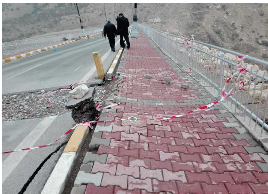
Figure 7. Cracks on Darbandikhan Dam crest, 2017
