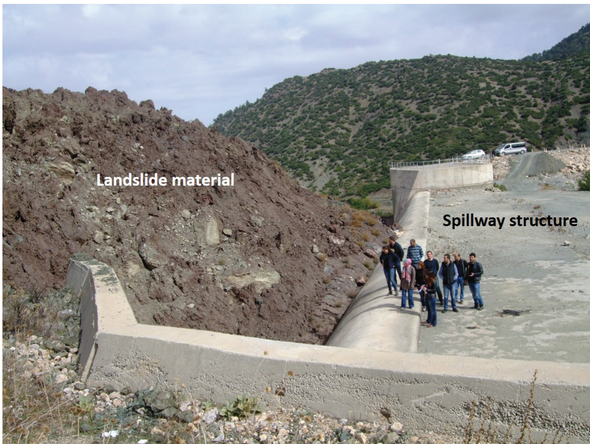
Figure 5. Landslide material in spillway structure area
