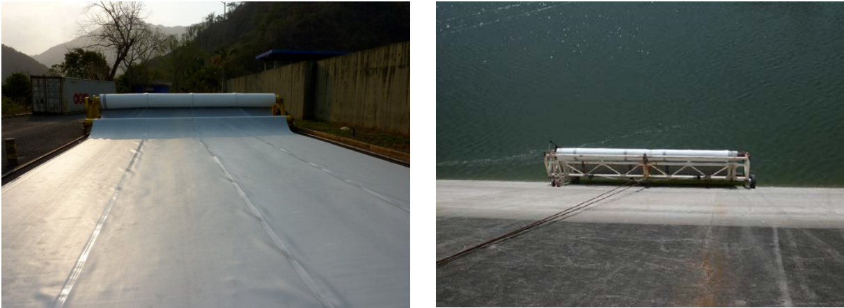
Figure 11. (Left) Prefabricated panel of SIBELON ® geocomposite, obtained heat-seaming four sheets, each with width of 2.10 m. (Right) Lowering of the pre-fabricated panel of SIBELON ® geocomposite in the water.
