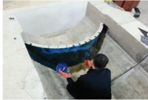
b) Application of MBT-MBrace®Adesivo to the body surface
