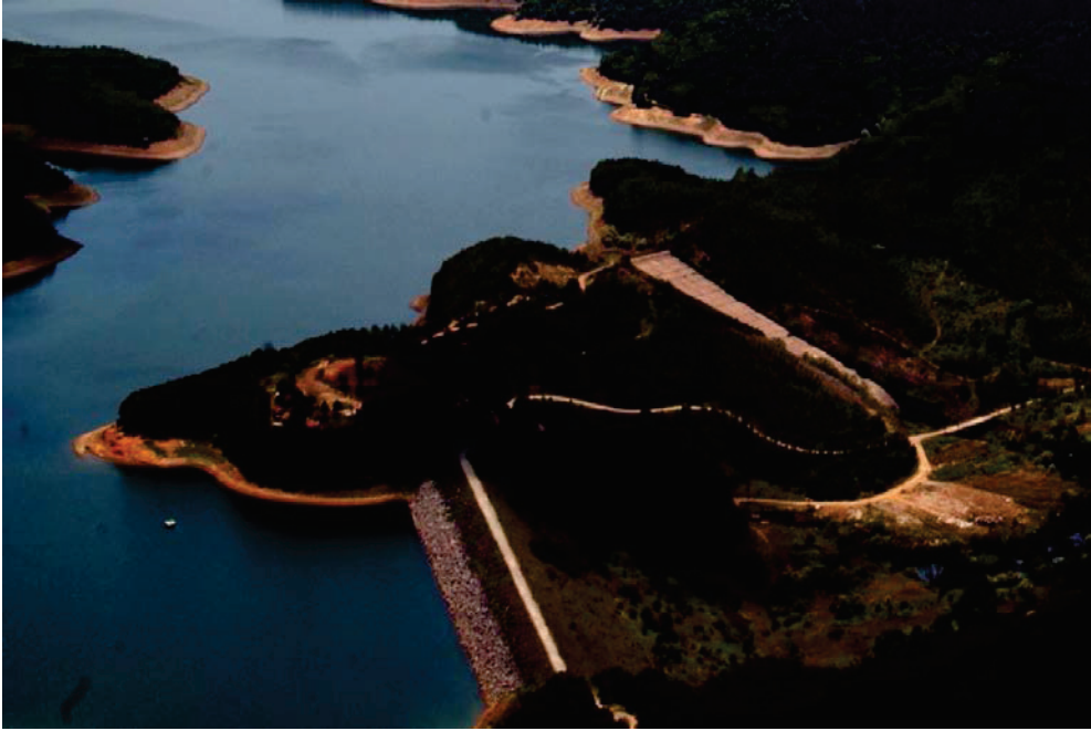
Figure 8. General view from Buyuk Cekmece dam.
