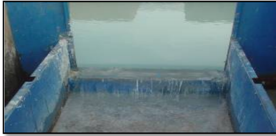
Figure 3. Spillway of thick wall tested (Model D1)
