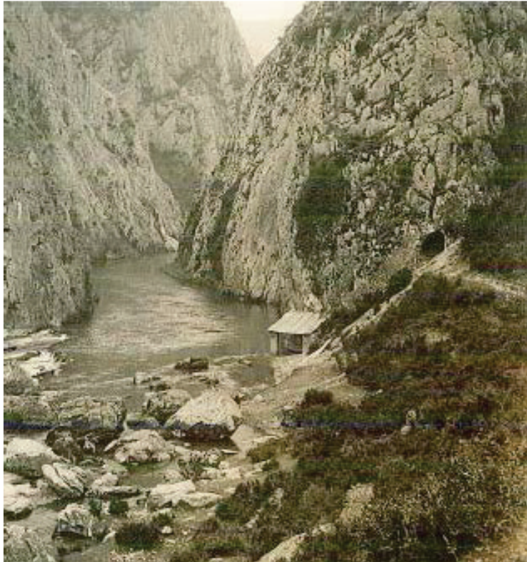
Figure 1. Canyon Matka on the river Treska in 1935, before construction of the arch dam
