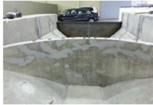
d) Application of structural repair mortar on the surface of dam arc
