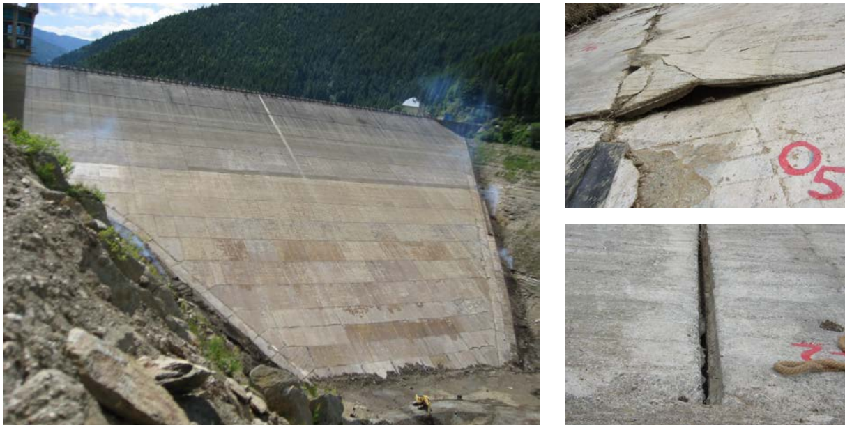
Figure 12. (Left) The upstream face of Pecineagu CFRD before installation of the SIBELON® geomembrane sealing system. (Right) Effect on concrete slabs and joints of the settlements in the dam body.
