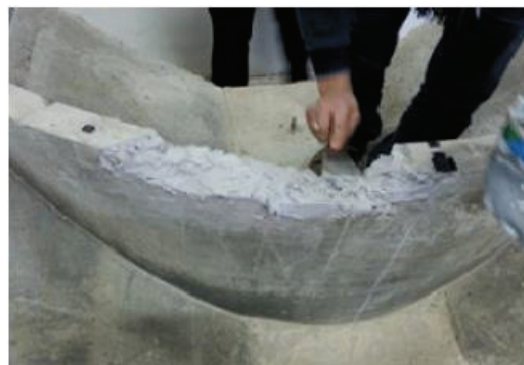
b) Application of structural repair mortar using hand trowelling proces
