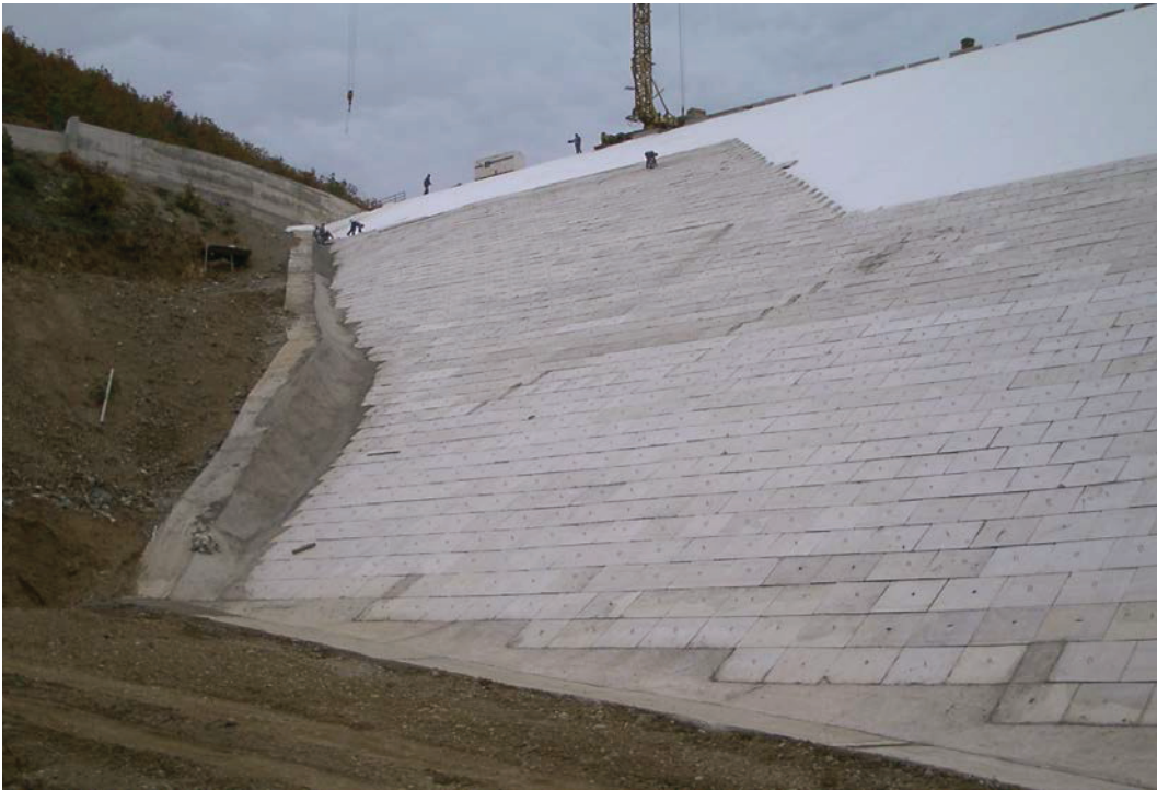
Figure 11. Rock-fill dam Loshana with geomembrane facing, built in 2006, Hs=45 m
