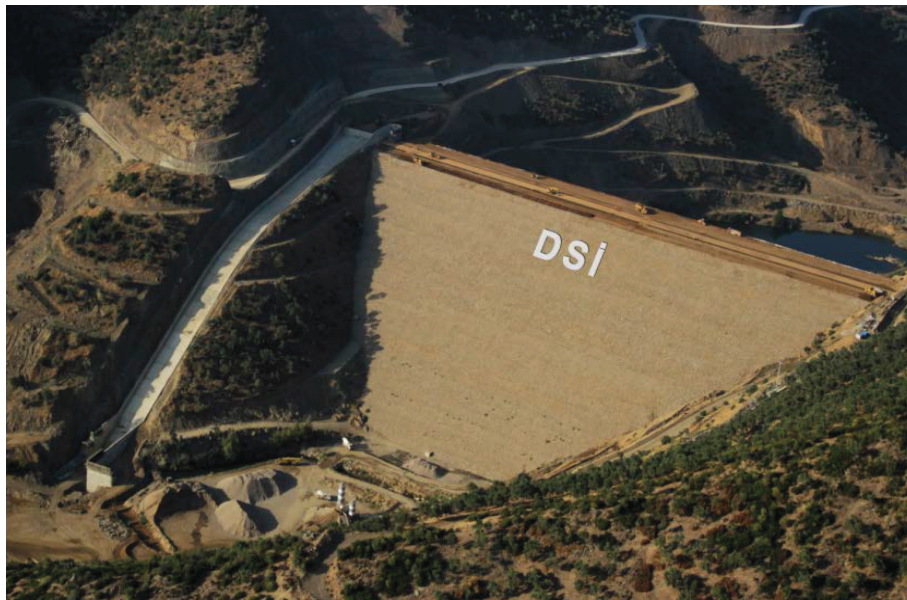
Figure 7. A general view from Burgaz dam.
