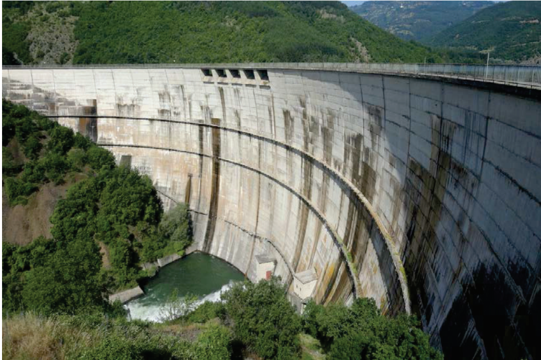
Figure 9. Lipkovo dam, constructed in 19672, the highest arch dam in R. Macedonia
