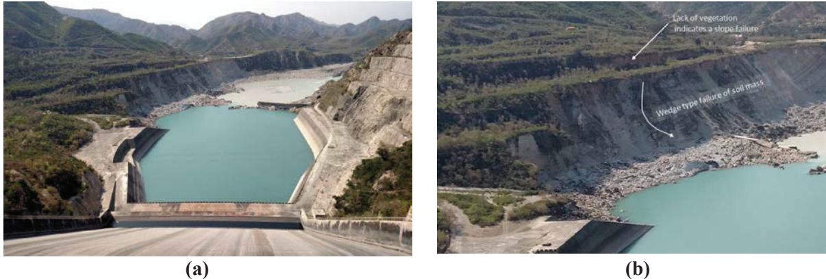
Figure 5. Erosion of slope on the Left-bank downstream of the Plunge Pool
