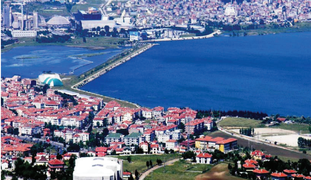
Figure 5. General view from Buyuk Cekmece dam.
