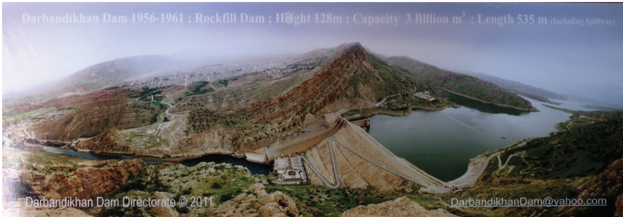
Figure7 . Darbandikhan (Derbendixan) Dam view of right bank
