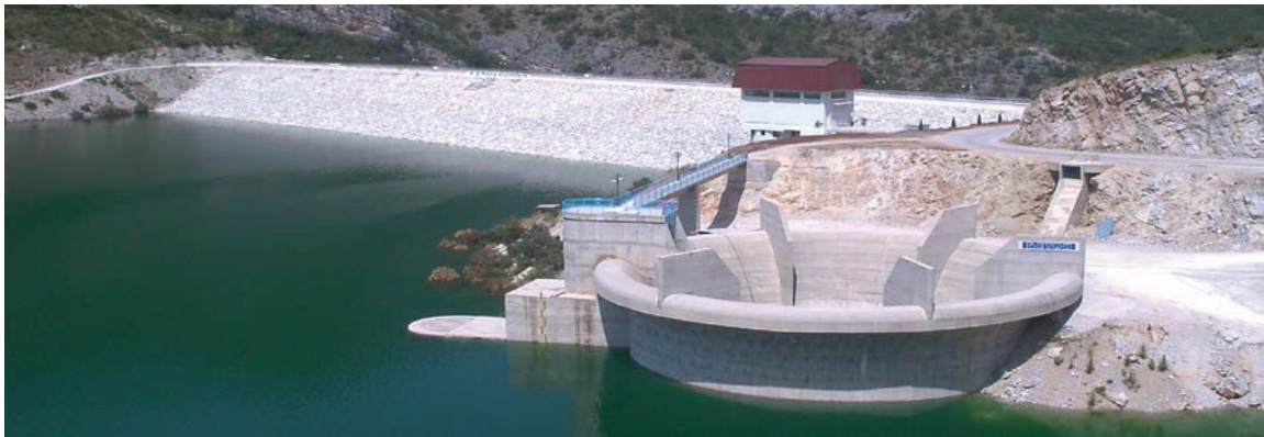
Figure 14. Upstream view of Kozjak dam, highest earth-rock dam in R. Macedonia
