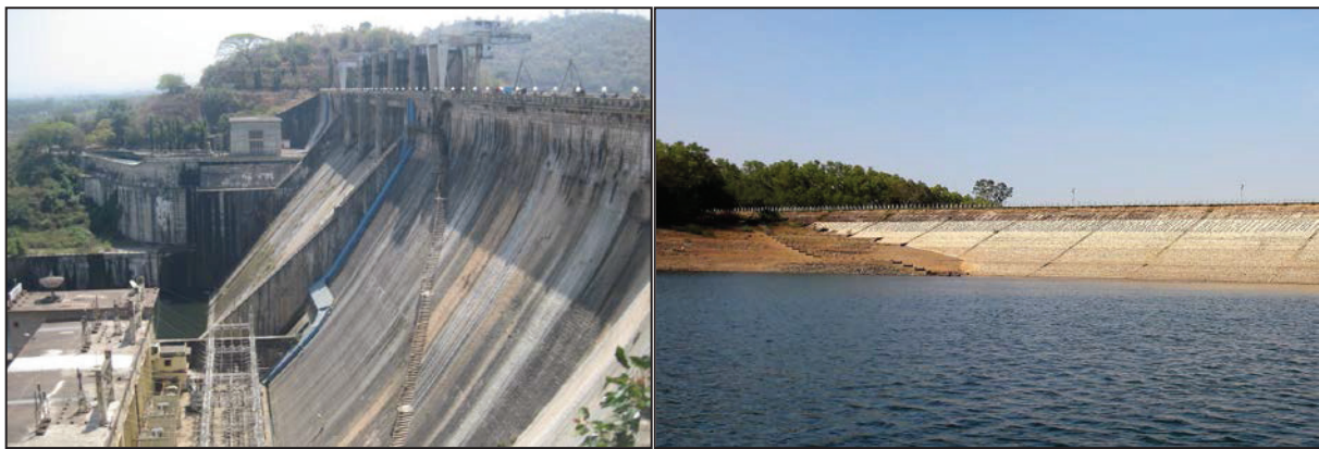
Figure 1. Bhadra dam-reservoir system. Left: masonry dam (back). Right: saddle dam (front)
