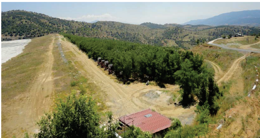
Figure 15. Tailings dam Topolnica of mine Buchim, with recultivated downstream slope
