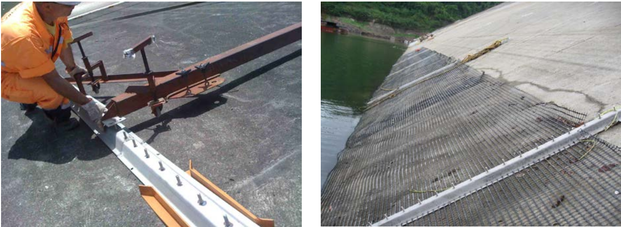
Figure 10. (Left) Detail of the tensioning profiles, customized for underwater installation. (Right) Geogrid installed between the tensioning profiles for supporting the waterproofing geocomposite.
