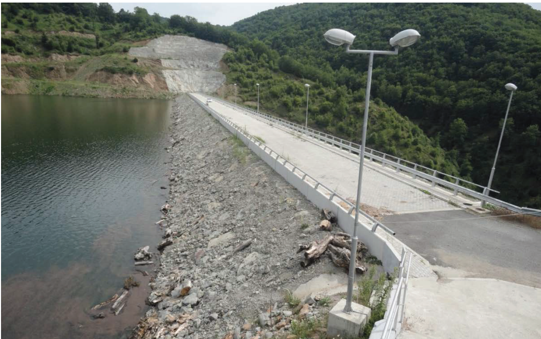
Figure 12. Rock-fill dam Knezevo with asphalt core, on river Zletovska, built in 2011, Hs= 82 m
