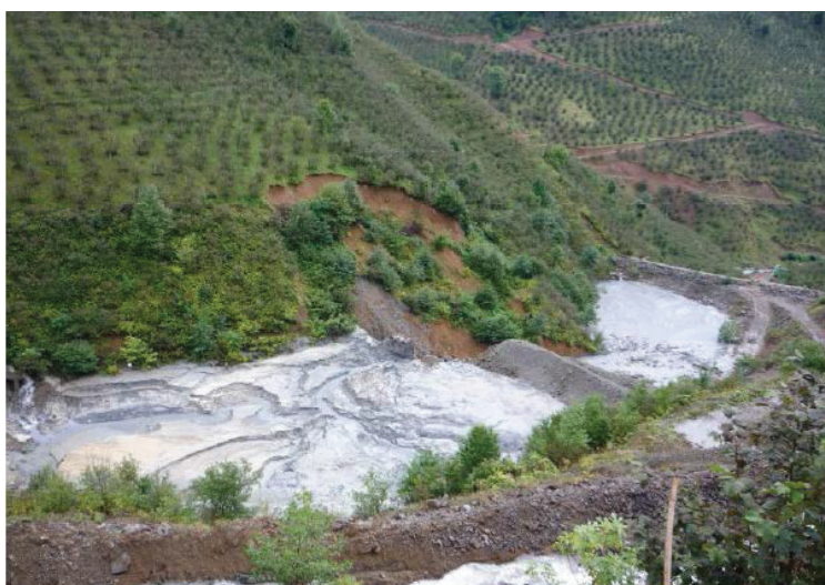
Figure 4. Tailings dam break in Ordu Province
