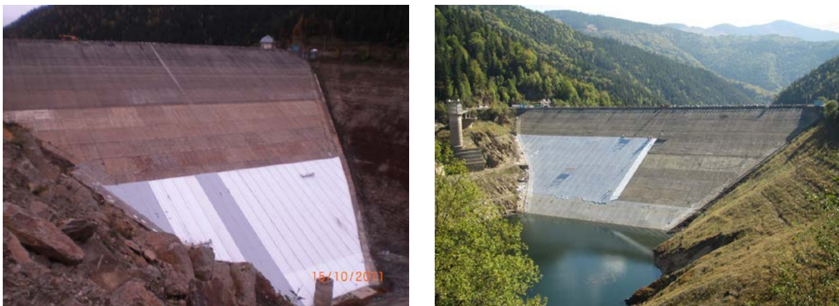
Figure 13. Waterproofing works ongoing during stage 1 (left) and stage 2 (right).
