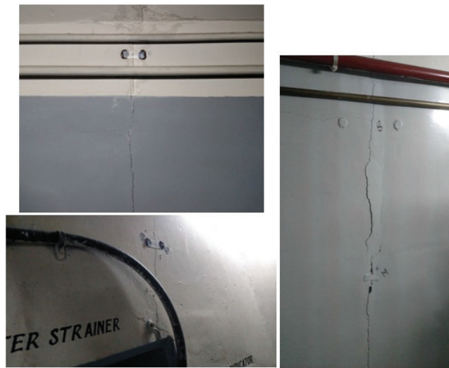
Figure 8. Cracks in the Turbine Pit of Unit-14
