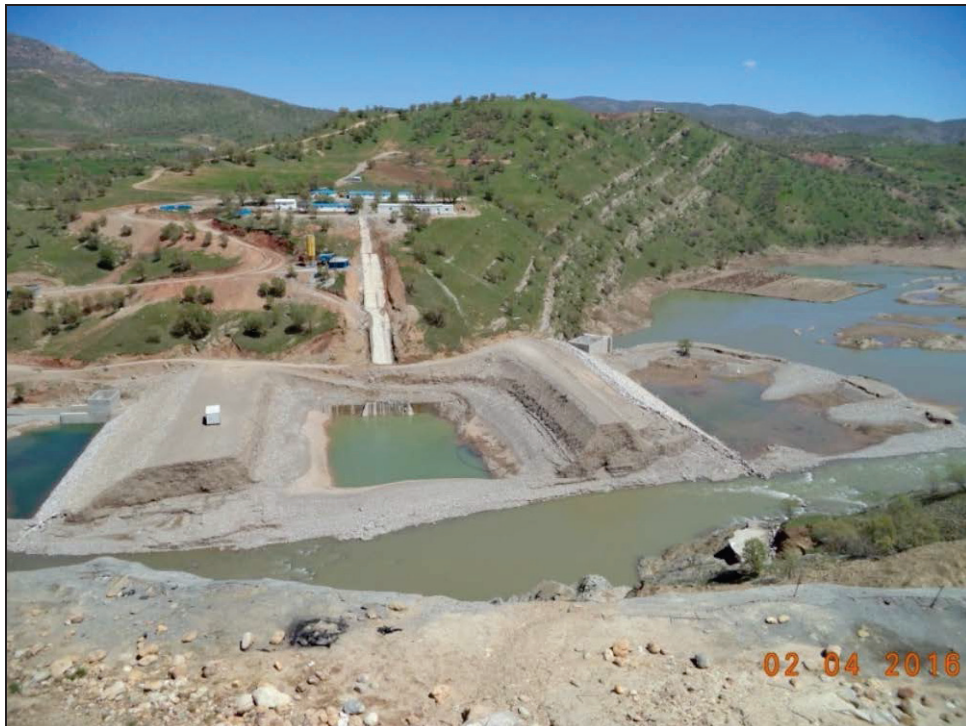
Figure 10 Harmn dam after the flood
