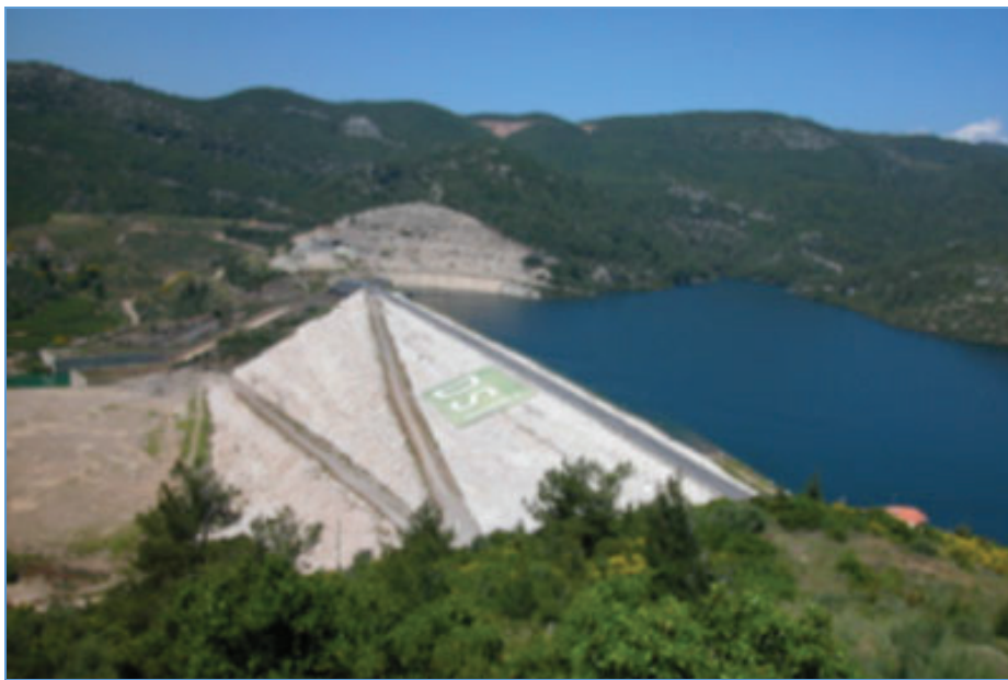
Figure 10. A general view from Tahtali dam
