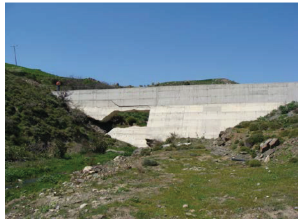
Photograph 4. Gennas Dam failure, 2014 (N. Moutafis, personal communication)
