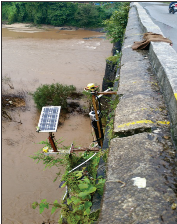
Figure 2. Measurement station at the river inlet into the Bhadra reservoir
