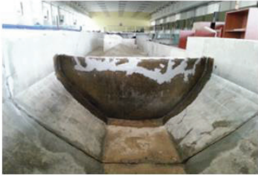
a) Application of MBT-MBrace®Primer to the body surface
