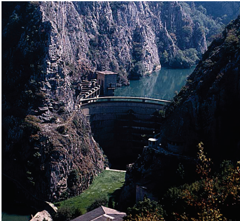
Figure 2. Downstream face of Matka dam, the first dam in R. Macedonia, built in 1938
