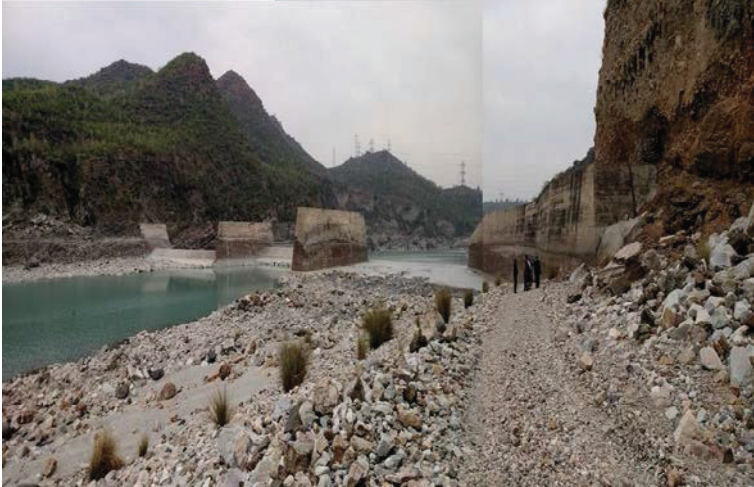
Figure 10. Panoramic view of Dal Darra Weir from Upstream Side
