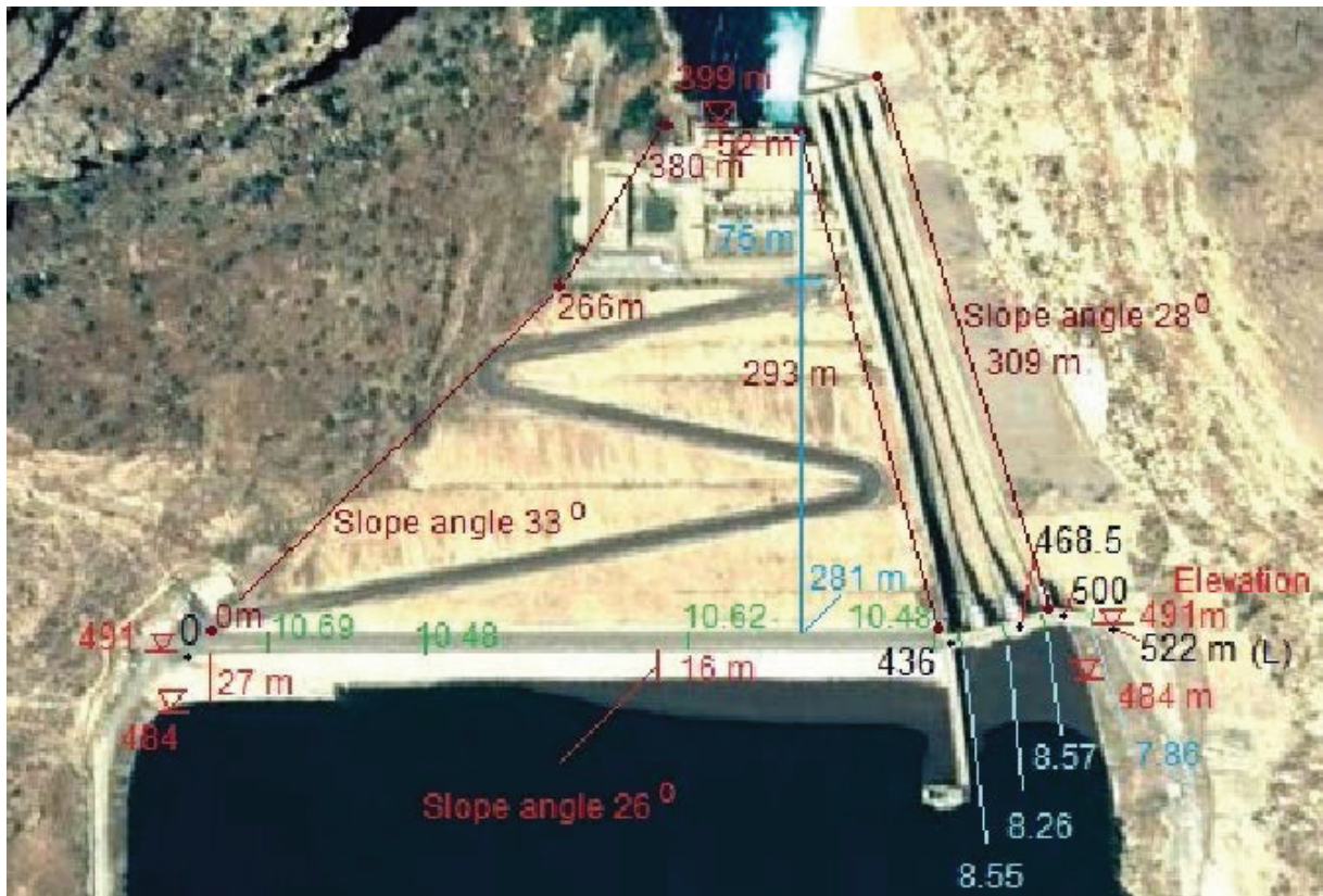
Figure 8. Darbandikhan Dam geometrical dimensions
