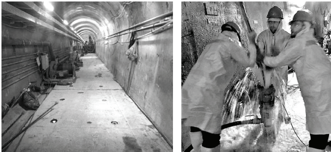
Figure 8. Gallery with Standpipes Cut Flush to Surface (left) and installation of packer through the preventer (right)
