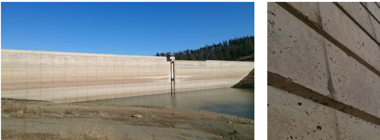
Figure 6. (Left) Upstream face of Grindstone Canyon RCC dam before the waterproofing works. (Right) Detail of the rustication joints in the conventional concrete facing.
