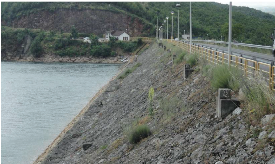
Figure 6. Upstream slope of Shpilje dam, constructed in 1969
