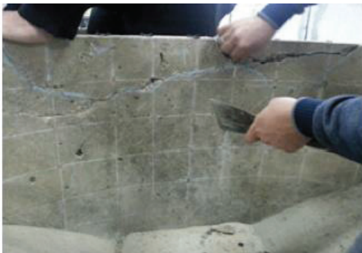
a) Removal of the damaged concrete pieces
