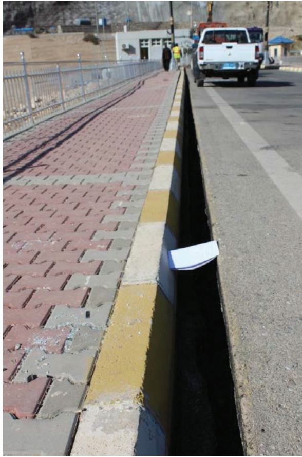
Figure11. Major downstream crack occurred on the Darbandikhan (Derbendixan) Dam
