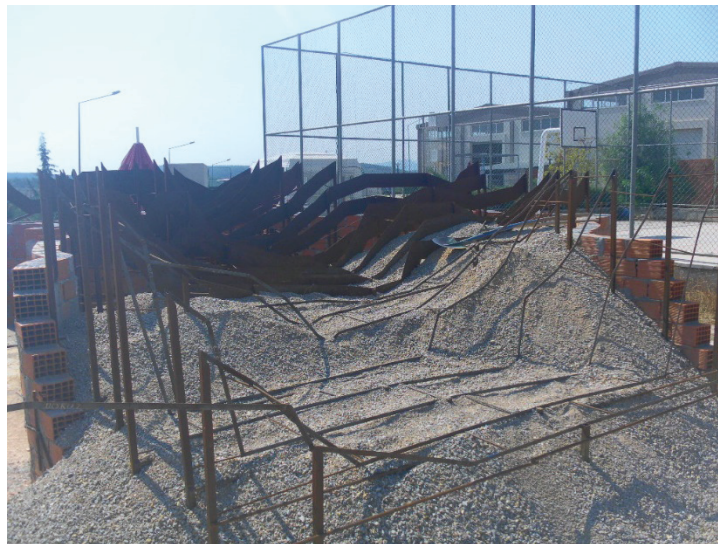
Figure 17. Filling granular material at dam reservoir
