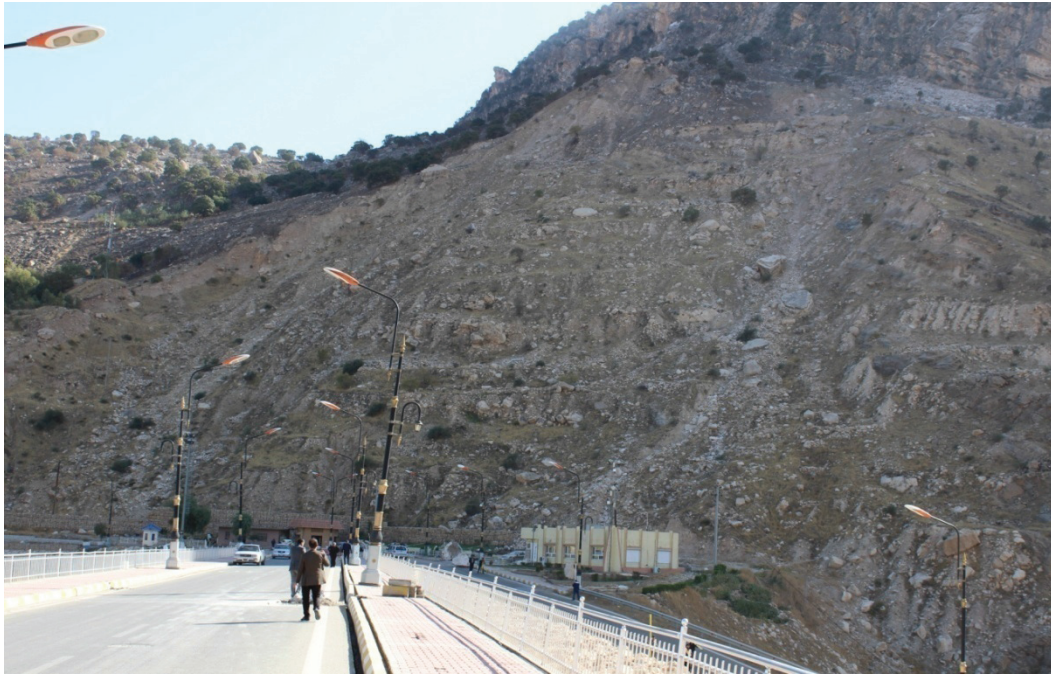
Figure 18. Active landslide occurred on the left bank of the dam and some fallen large blocks
