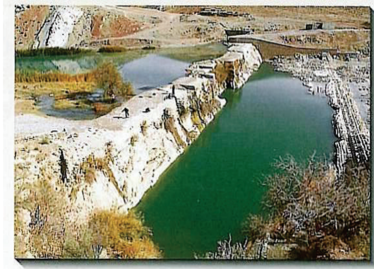
Figure 3. Bahman Dam in Iran
