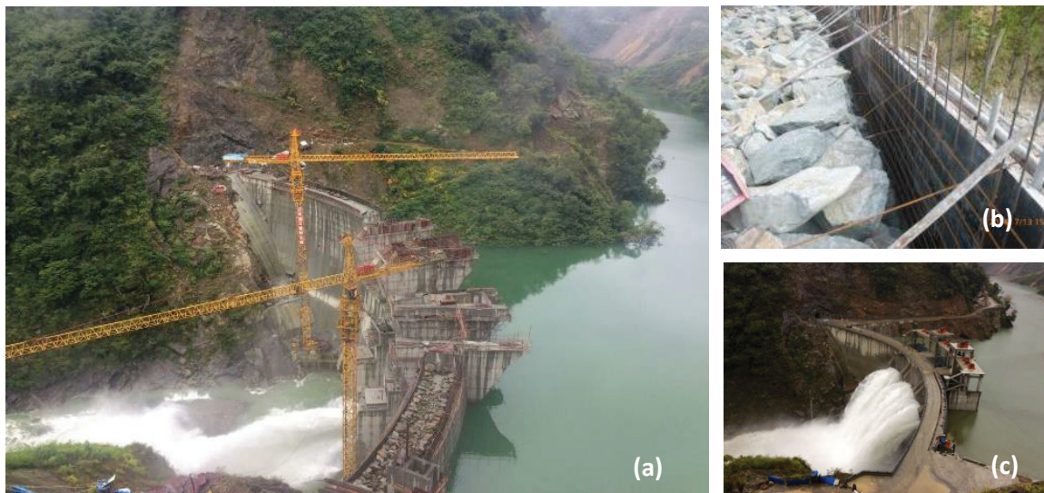
Figure 2. (a) The Baijia RFC double-curvature arch dam (H = 69 m) under construction, (b) the impermeable layer before HSCC is poured, and (c) the photo taken after construction completed
