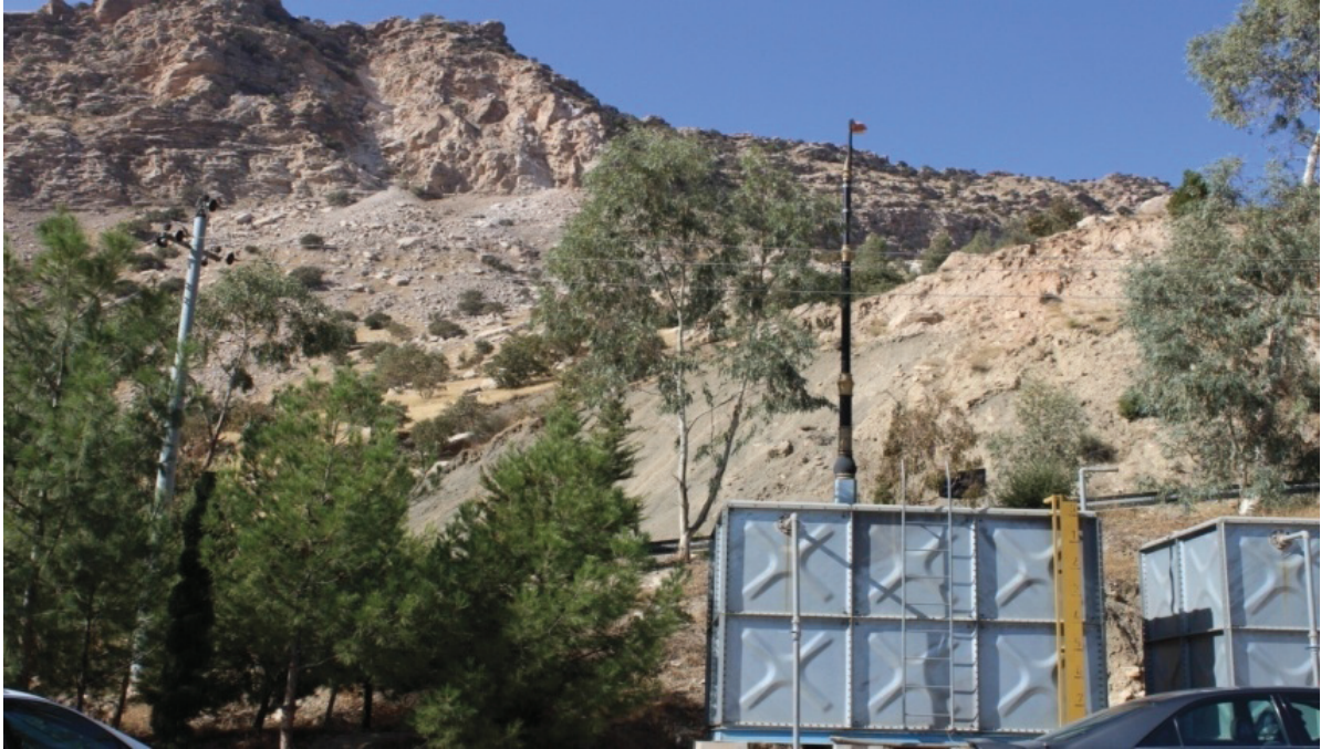
Figure 14. Unstable and loose rock blocks on the slopes of right bank of Darbandikhan dam
