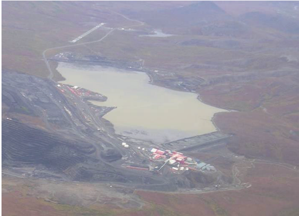
Figure 16. Tailings aerial photo
