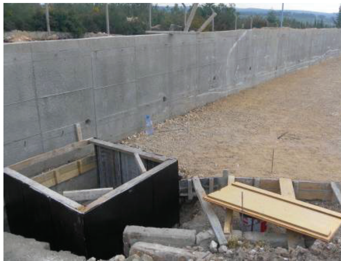
Figure 10. Canal and drainage hole for draining surface water
