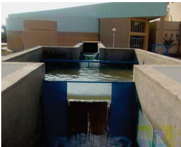
Figure 2. Reservoir test facility
