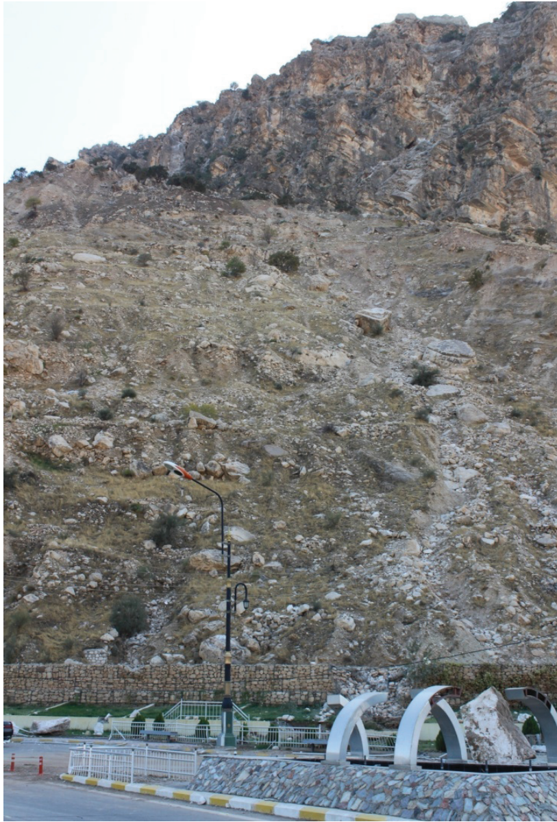
Figure 17. Some very large limestone blocks on the left bank of the dam which became unstable and fallen
