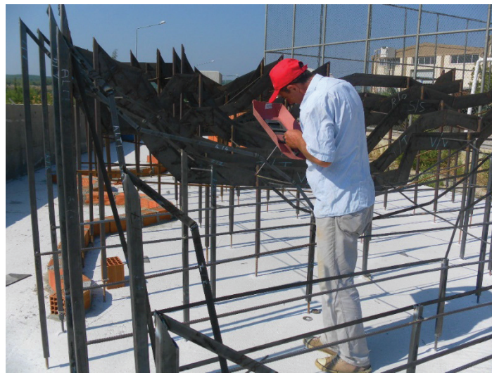
Figure 15. Placement of metal sheets for dam reservoir
