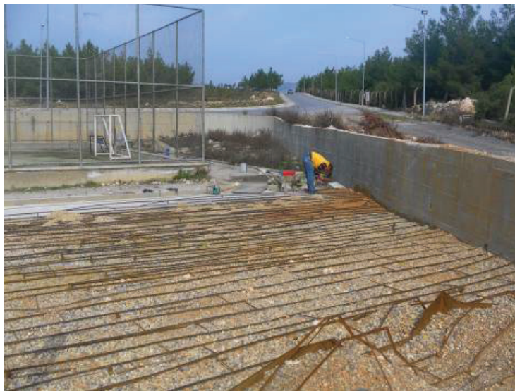
Figure 21. Filling granular material before concrete pouring
