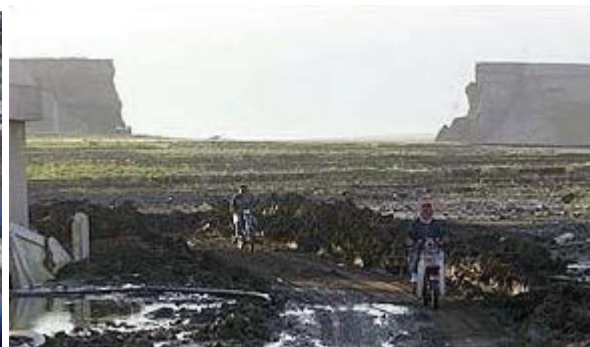
(b) Remaning Part of Dam Body
