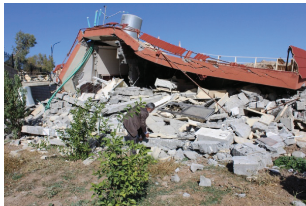
Figure 15. A ruined structure on the right bank of Darbandikhan (Derbendixan) dam
