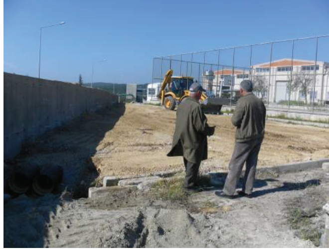
Figure 9. Leveling ground
