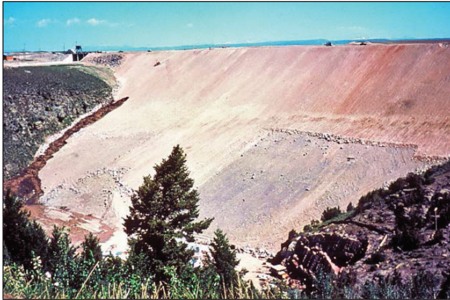
Figure 1: Teton Dam Failure
