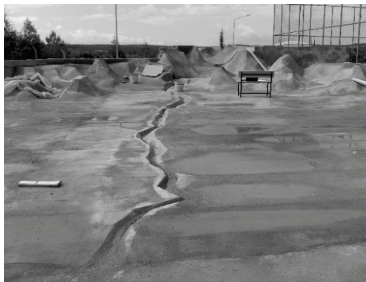
Figure 24. Downstream topography and the Creek view
