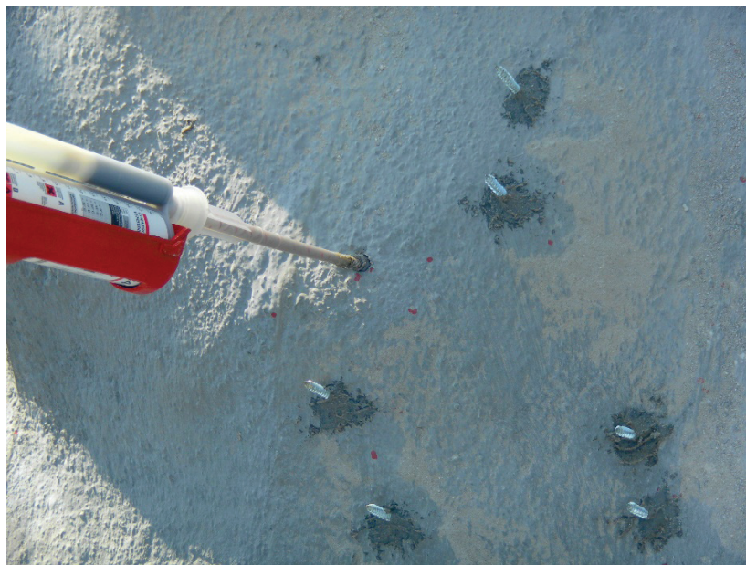
Figure 26. Screws prepared for mounting buildings
