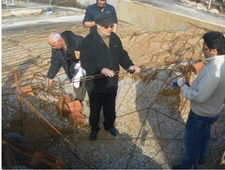
Figure 20. Placement of metal bars cross sections
