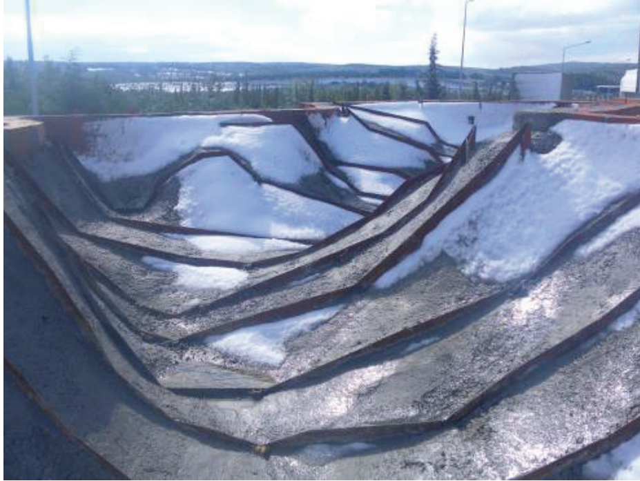
Figure 18. Pouring concrete at dam reservoir
