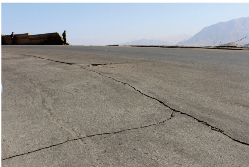
Figure 13. View of the cracks in the road owchic is on the right bank of Darbandikhan Dam
