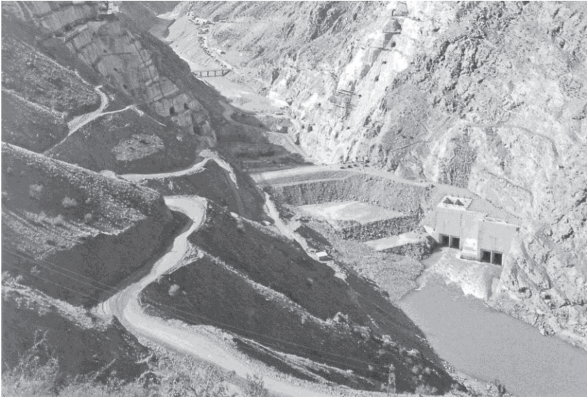
Figure 4: Intake portals of diversion tunnels of Karakaya Dam (Turkey) during construction (Hydraulic Engineering Works Italstrade: Milan 1990)
