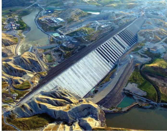
Figure 1. General view of Ilisu dam (DSI 2018).
