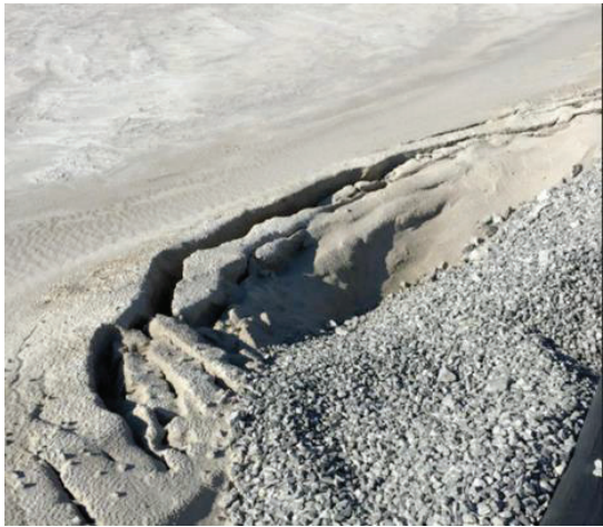
Figure 6. Sinkhole in new tailings
