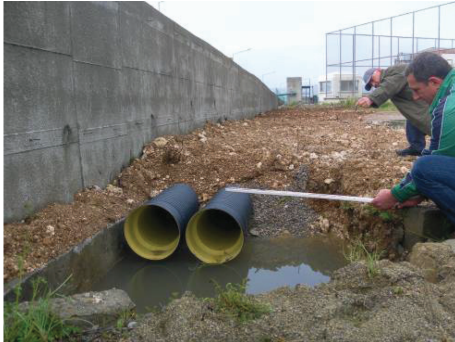
Figure 8. Placement of drainage pipes
