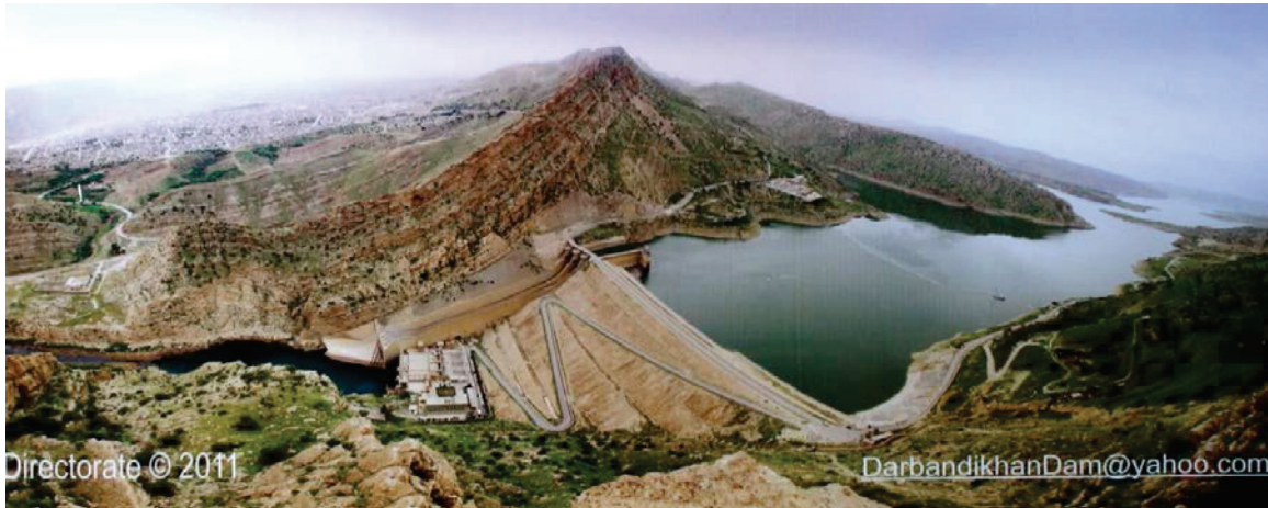
Figure 12. Darbandikhan (Derbendixan) Dam view of right bank
