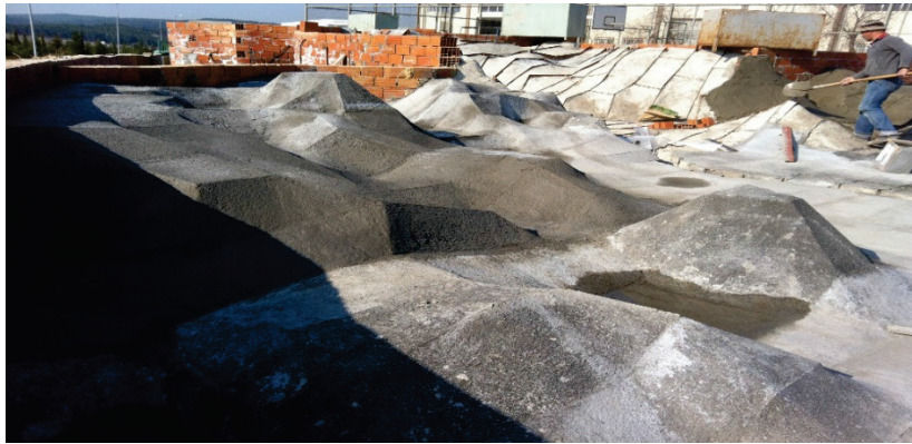
Figure 23. Leveling surface
