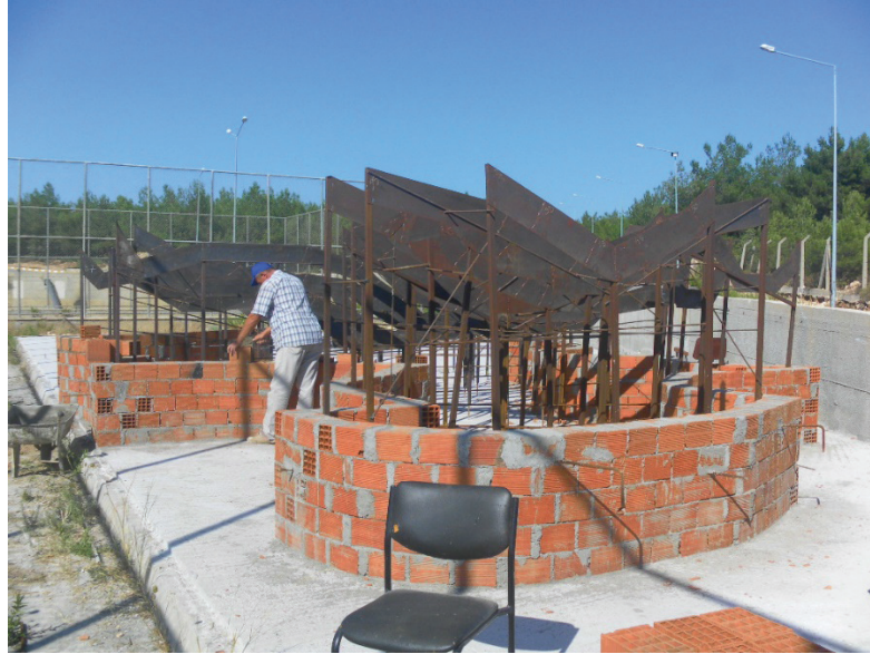
Figure 16. Construction of brick wall around the dam reservoir
