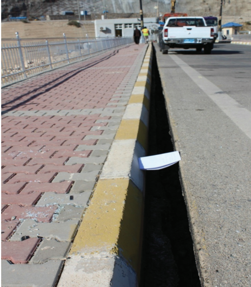
Figure16. Major downstream crack occurred on the Darbandikhan (Derbendixan) Dam
